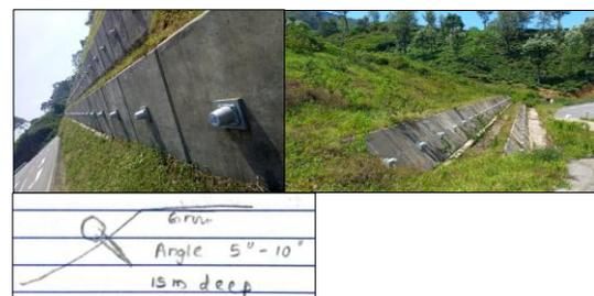
Figure 6. Ground anchors
