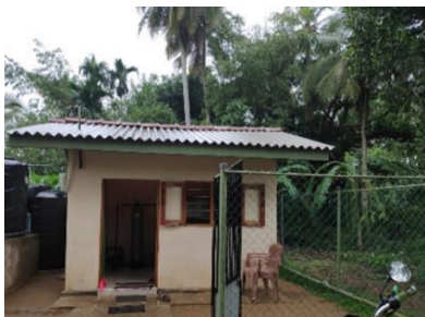
Figure 4. BWRO Facility building
