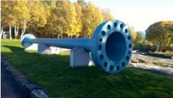
(b) Figure 1. Bergsøysund Bridge: (a) the bridge and (b) flexible rod
