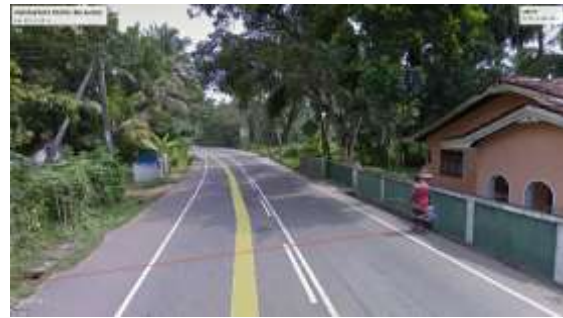
Figure 7 (Tangalle Road Cutting)
