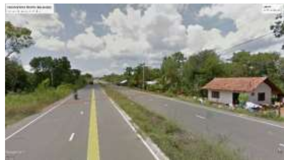
Figure 8 (Kiriebanara-Sooriyaweaw Road Cutting)
