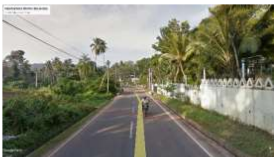
Figure 5(Dikwella-Beloatta Road Cutting)
