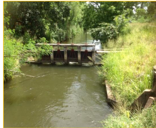
Figure 4: Left bank canal with water control unit of Rajanganaya 5km away from the dam
