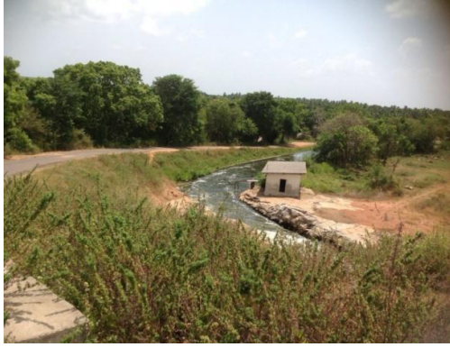
Figure 3: the left bank canal just below the sluice outlet
