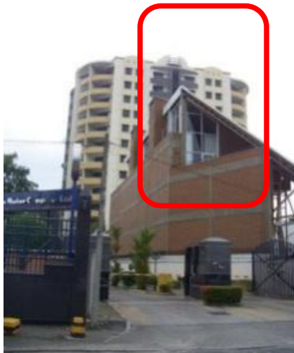
Figure 4: Thermal Chimneys in Case Study One
