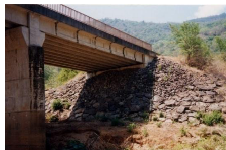
Figure 15 : Kurundu Oya Bridge
