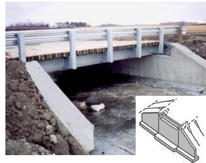
Figure 4: Typical applications of straight wing walls
