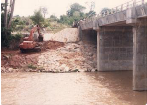
Figure 16: Badulu Oya Bridge
