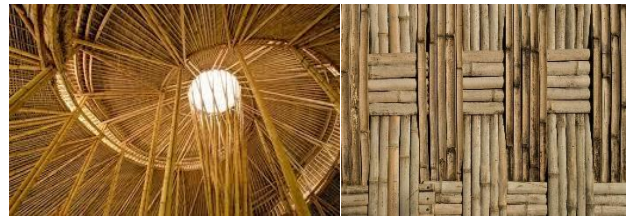
Figure 8: Bamboo as construction material (a) Roof and columns (b) walls
